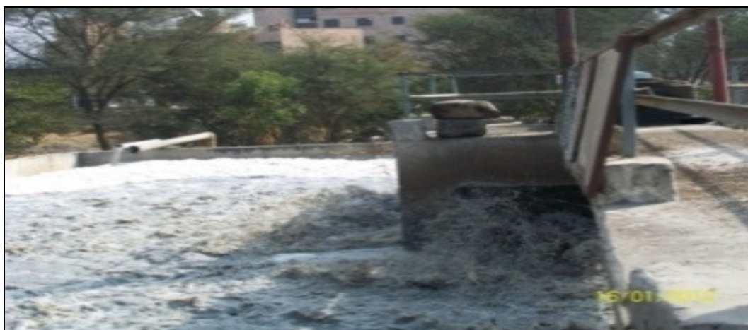
Fig.-2: Effluent (Aeration Tank) Jaipur Dairy
